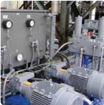
For hydraulic systems, the PLC logic manages the hydraulic power unit circuits to only allow hydraulic pressure to the appropriate unheading valve when the process is verified safe. Additionally our high-performance hydraulic power unit incorporates redundant equipment such as pump trains, and filters to maximize reliability. The hydraulic circuit is fully instrumented to provide real time status and includes alarms to facilitate preventative maintenance for a longer lasting robust system.
