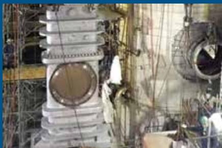
FCC Reactor Isolation
